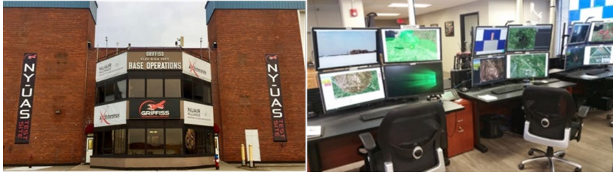
Figure 15: NUAIR base operations building at the Griffiss International Airport (left), along with the operations command center work stations (right). Source: NUAIR https://nuair.org/photos/
