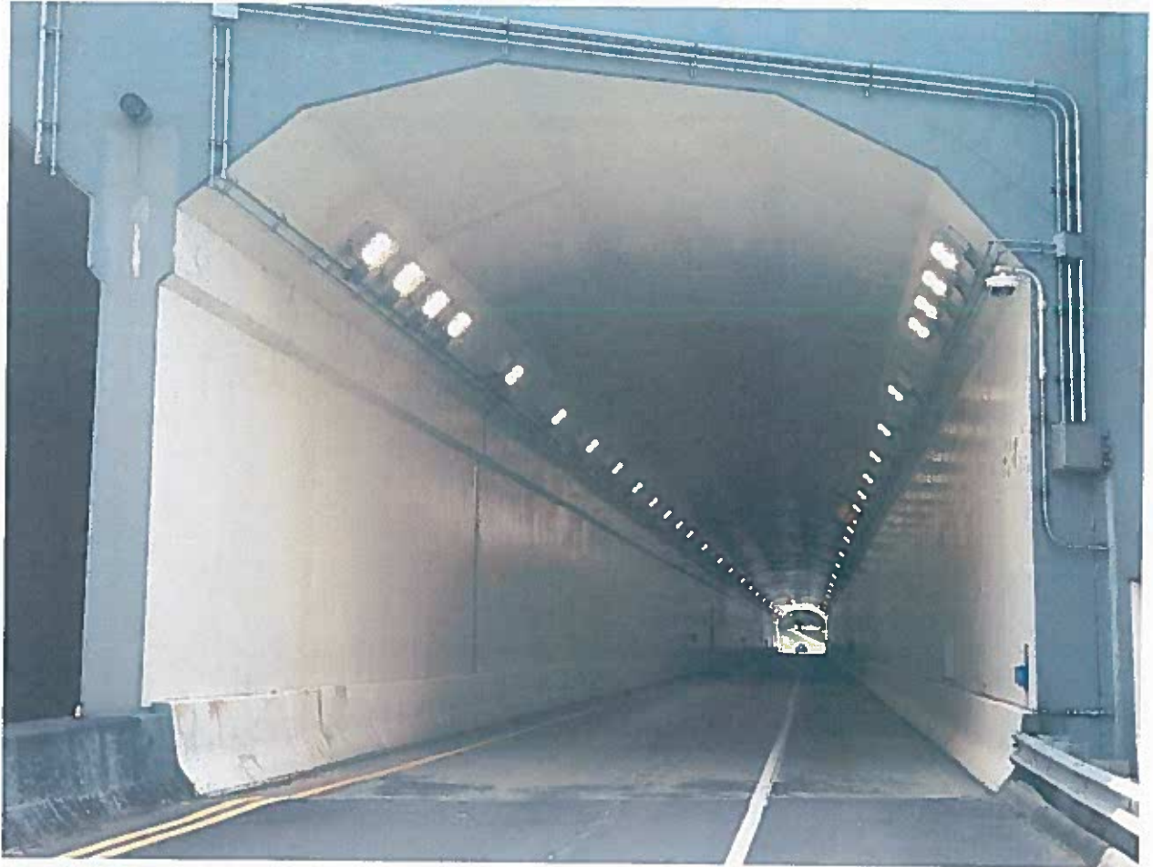
RWY 24 Tunnel Inspection
